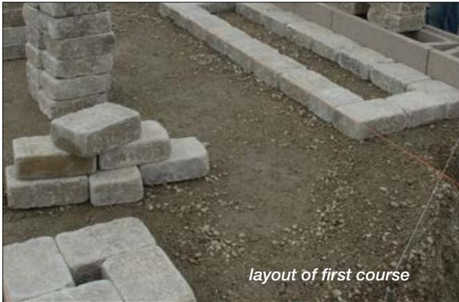
Lay out the entire first course and level each stone front to back, side to side, and stone to stone. Use a plastic dead-blow hammer as necessary to make small adjustments.
