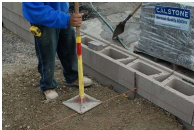
The soil beneath the base material must be firm and stable. If soil is soft, replace it with additional compact baserock.
