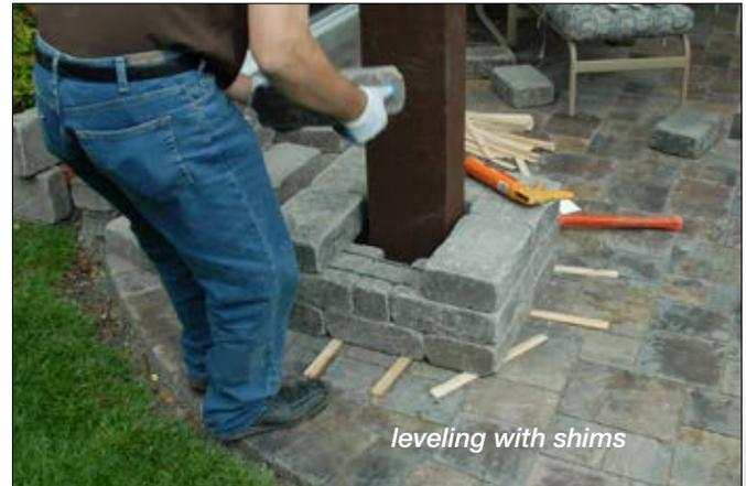
Leveling adjustments can be made by shimming with thin pieces of wood, ceramic tile wedges, or other devices to hold the first course level until the adhesive sets up.
