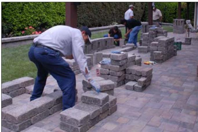
Interlocking pavers should be on a compacted base at least 4" thick. The width of any pavement should allow full contact for the first course of the Roman Stone. This will ensure good stability for your project.
